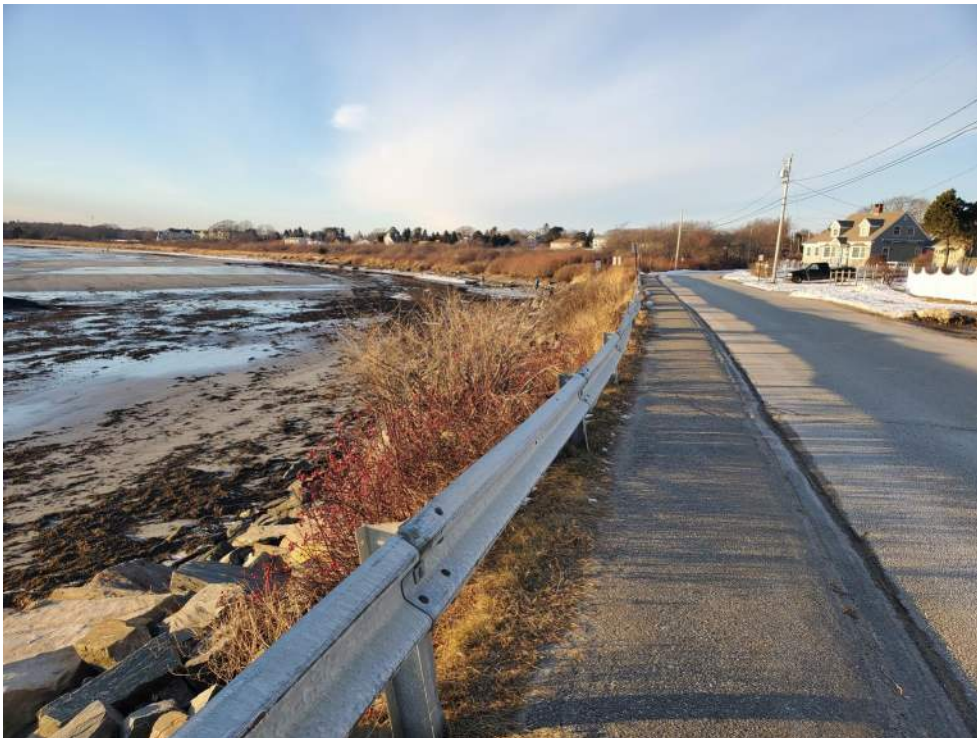
Photo 2 (01/09/2020): Kettle Cove Road and sidewalk with existing metal guardrail.
